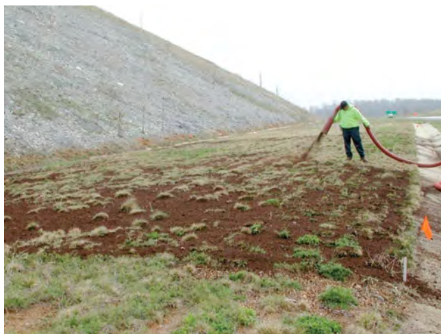
Figure 9.12. Applying compost to highway roadside to revegetate poorly established turfgrass. Photo courtesy of Greg Evanylo.
