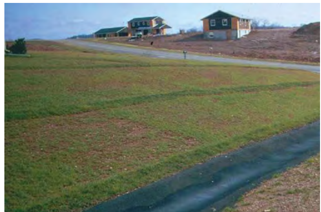
Figure 6.13. Adding single strips of sod to seed establishments on sloped sites is a highly effective means of reducing soil erosion potential.
