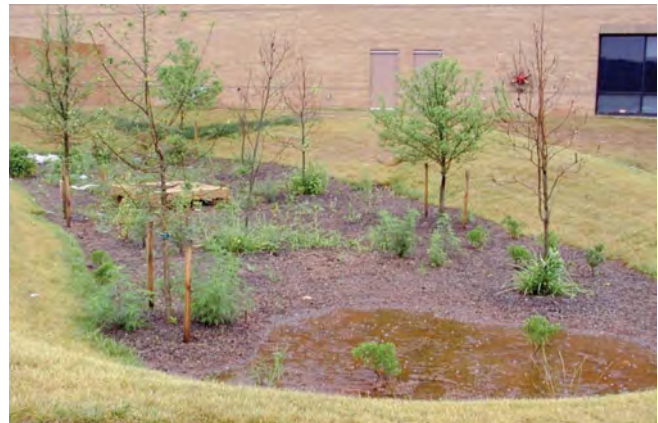
Figure 9.8. Bioretention rain garden.
