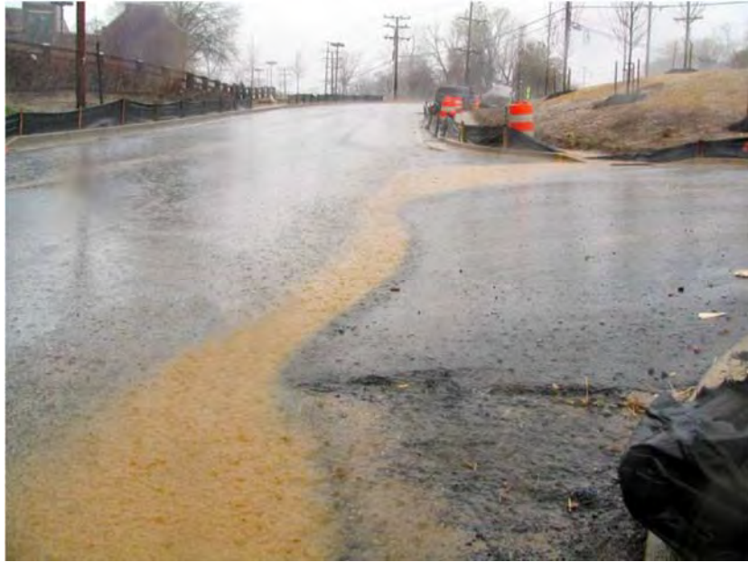
Sediment from Construction Runoff
